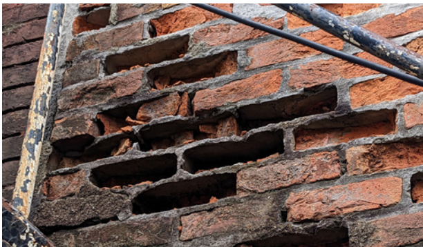
Example of deterioration to masonry caused by inappropriate strength mortar repair
